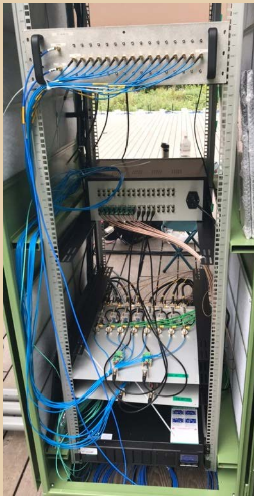
with housing and 16 balun boards
